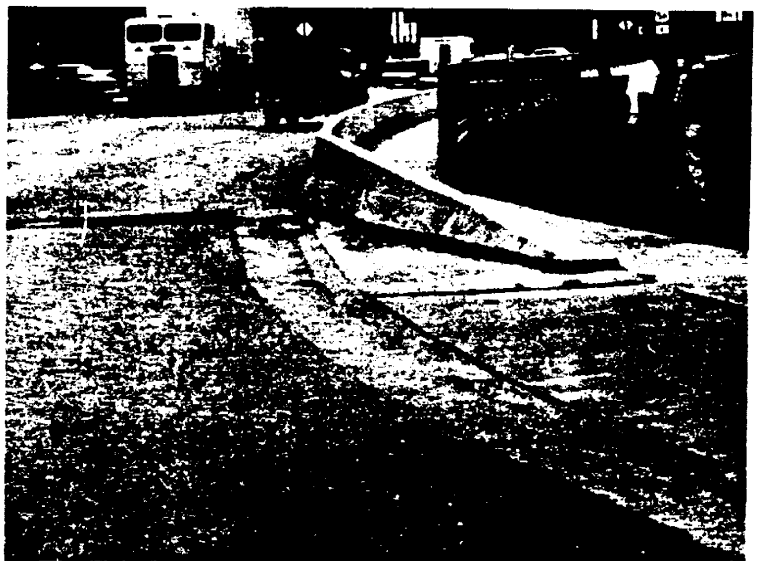
Figure 5-15. Barrier end treatment for speeds of less than 50 km/h.
