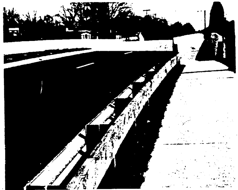
Figure 5-5. Protective rail on the backside of a guardrail adjacent to the sidewalk.
