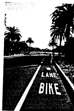
Figure 3-7. Example of a bike lane in Honolulu, Hawaii with text and arrow. (Source: www.pedbikeimages.org/Dan Burden)
