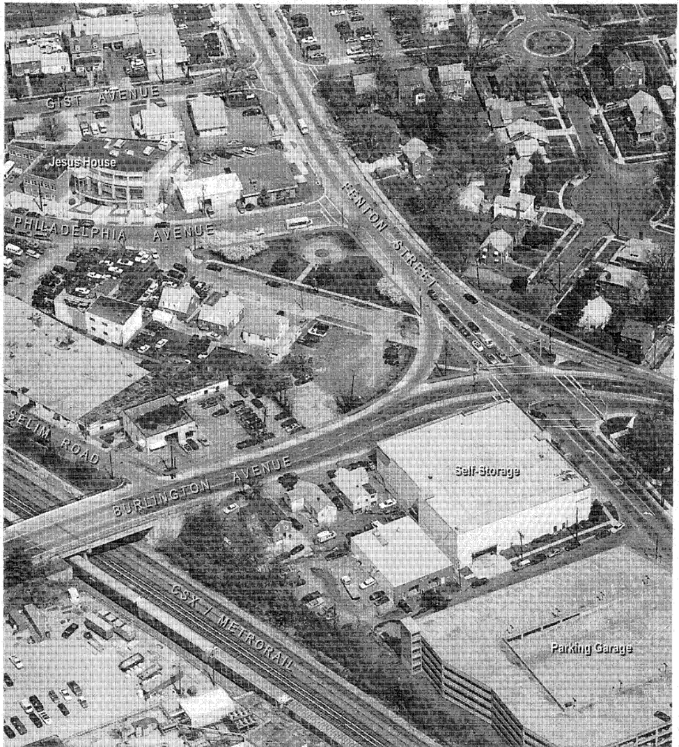
View to the North
