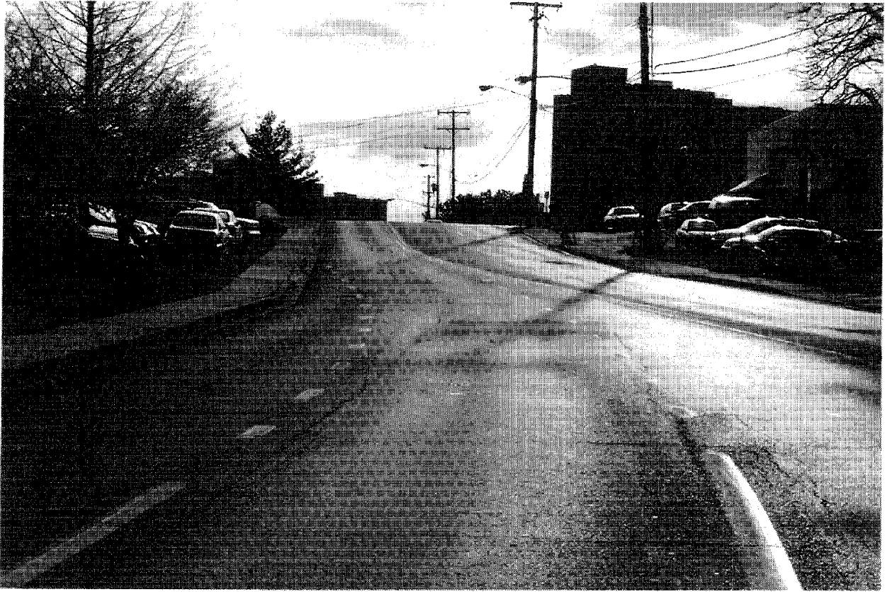
Photo 2. Burlington Avenue (MD 410) westbound from intersection with Fenton Street.
