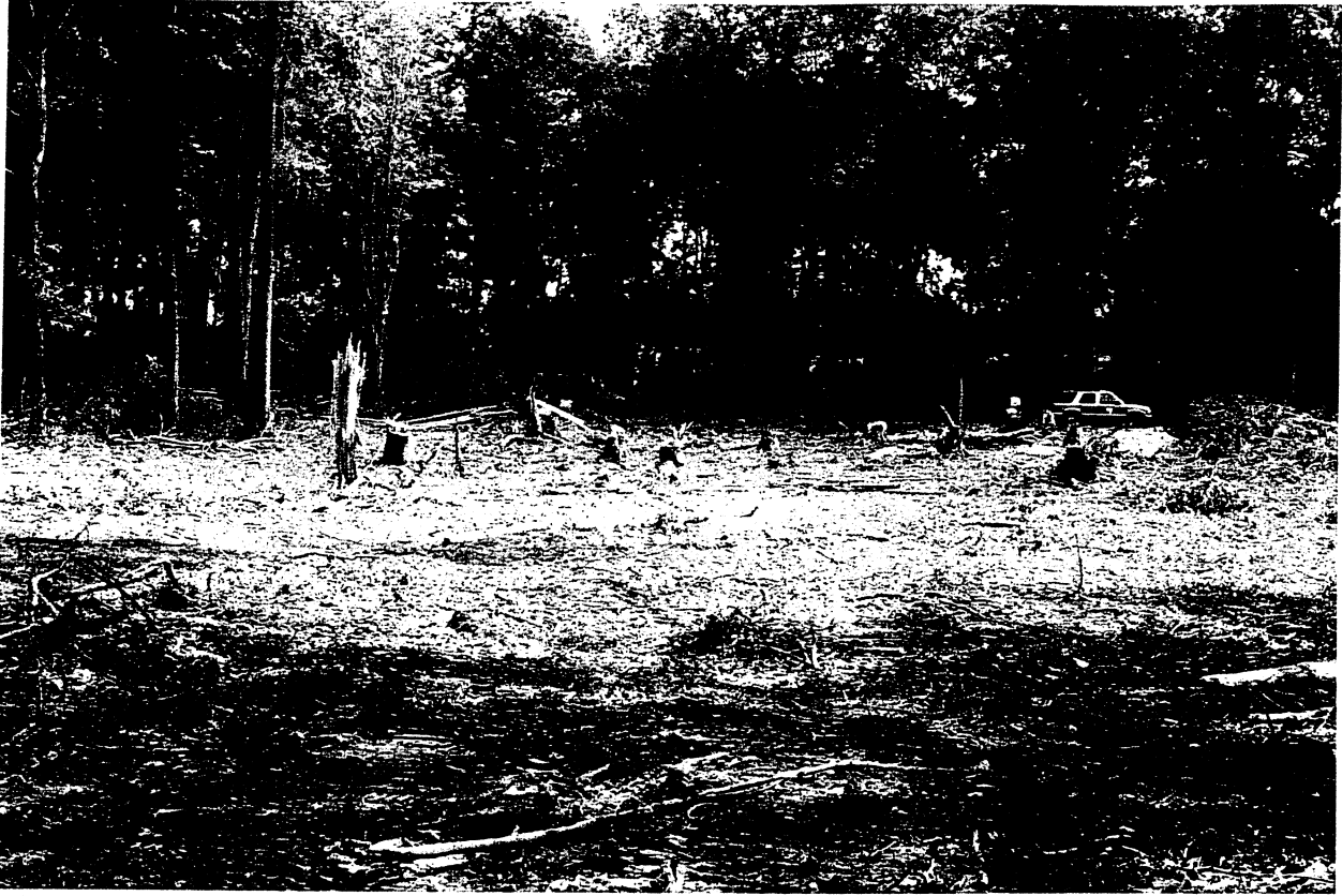
View from back of lot out toward Trundle Road showing cleared area. Note 555 Tracked Loader marks in near foreground.
