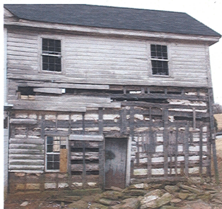
West block, north facade
