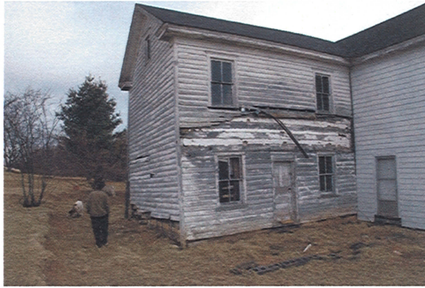
West block, south facade
