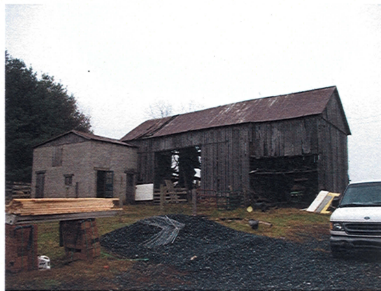
Barn, looking northwest
