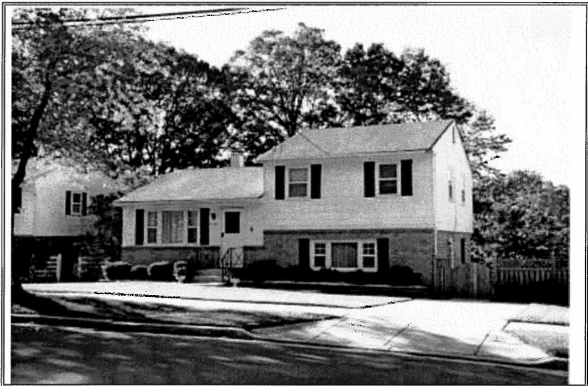
Plate 18: Split-level House (6816 Elbrook Road, Good Luck Estates, Prince George's County)
