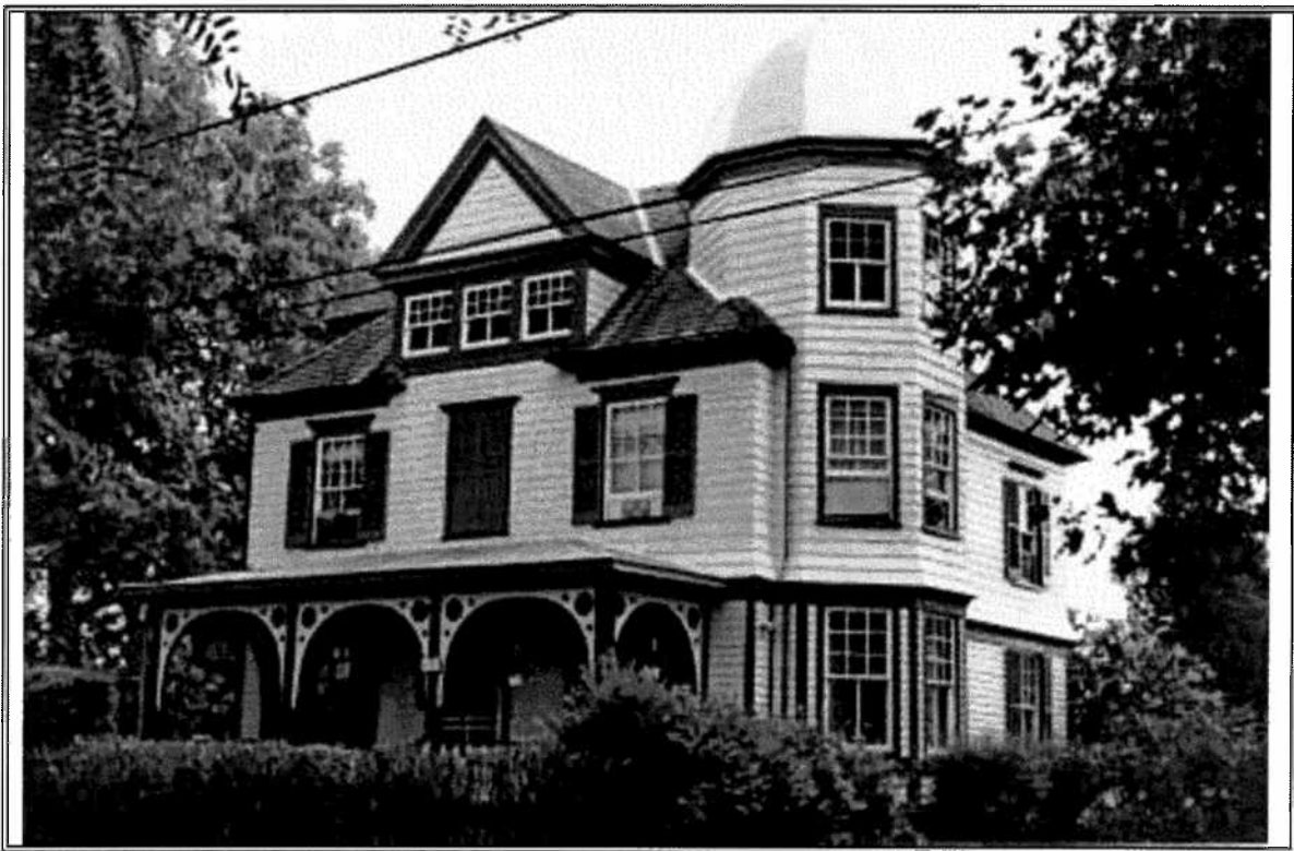
Plate 9: Queen Anne (4900 block of Oliver Street, Riverdale, Prince George's County)
