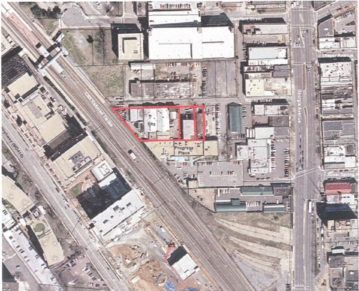
Site Aerial View
