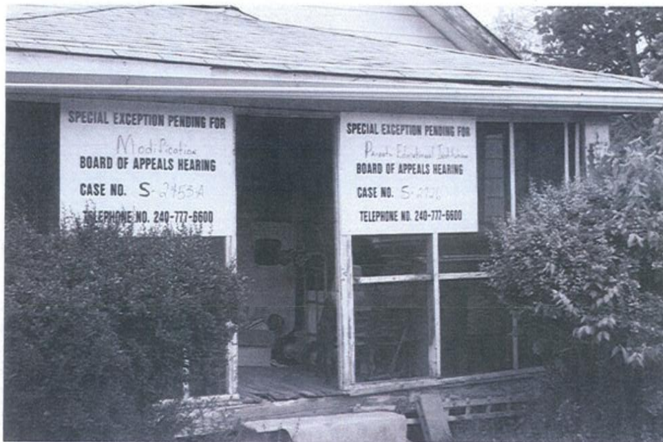
Figure 4: Existing house (vacant, used for storage)
