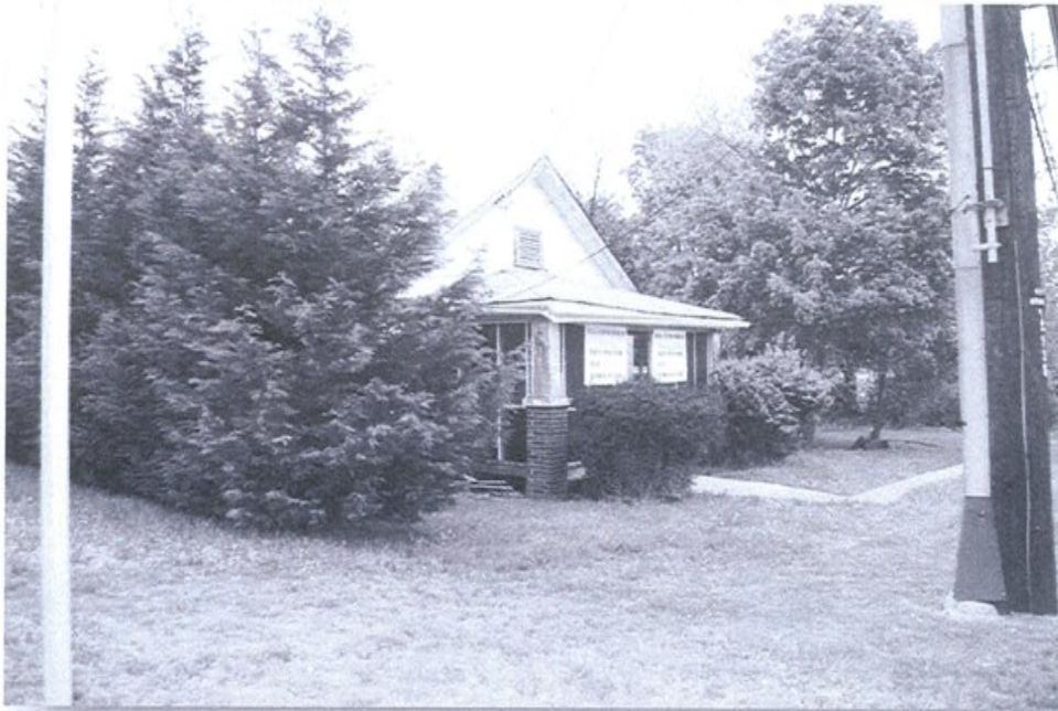
Figure 5: Existing House (to be demolished)
