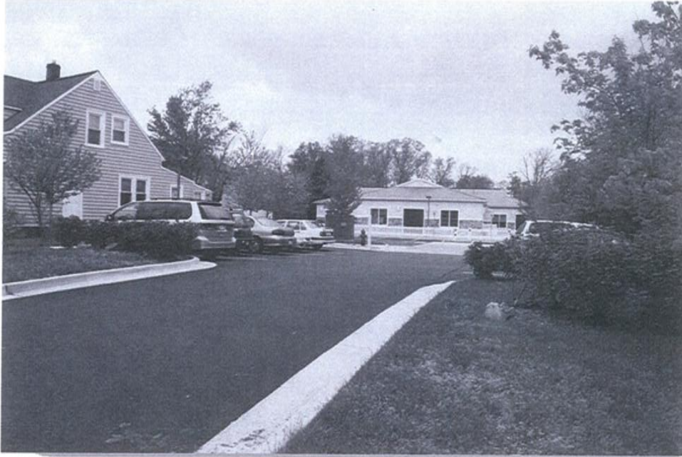
Figure 1: Site looking from Darnestown Road, north. Existing buildings.
