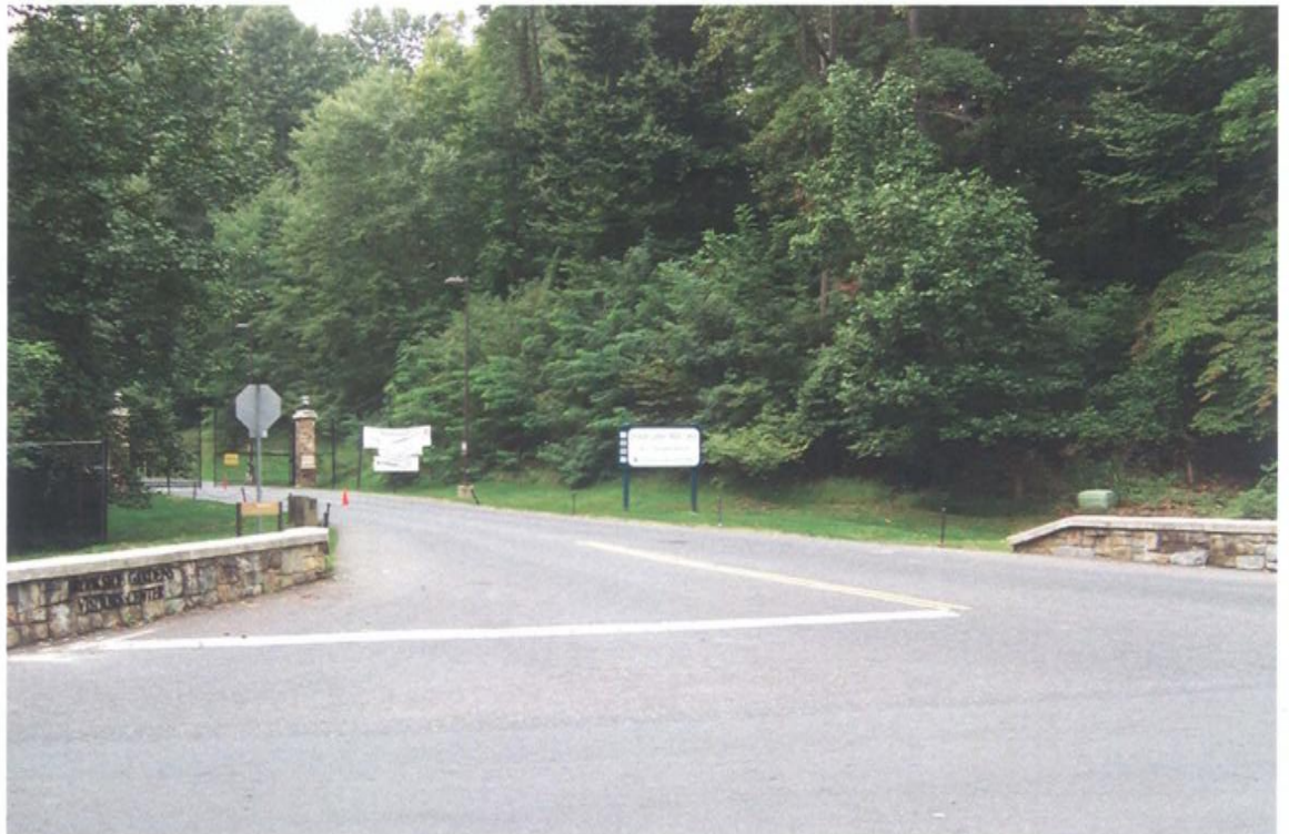
Existing entry road at bridge
