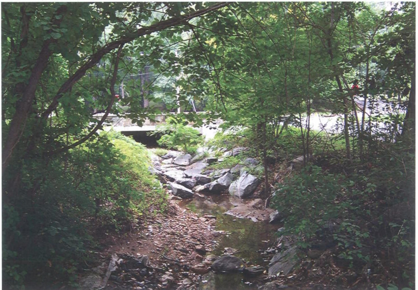
Glenallan Tributary, looking west towards bridge
