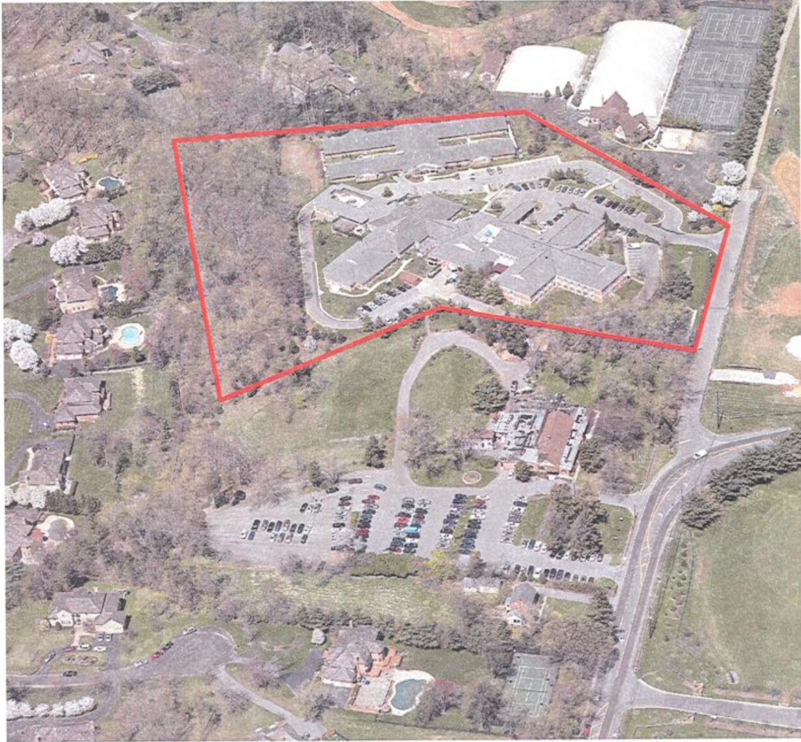
Aerial Photo (looking south)
