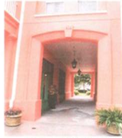
PORTICO TO COURTYARD
