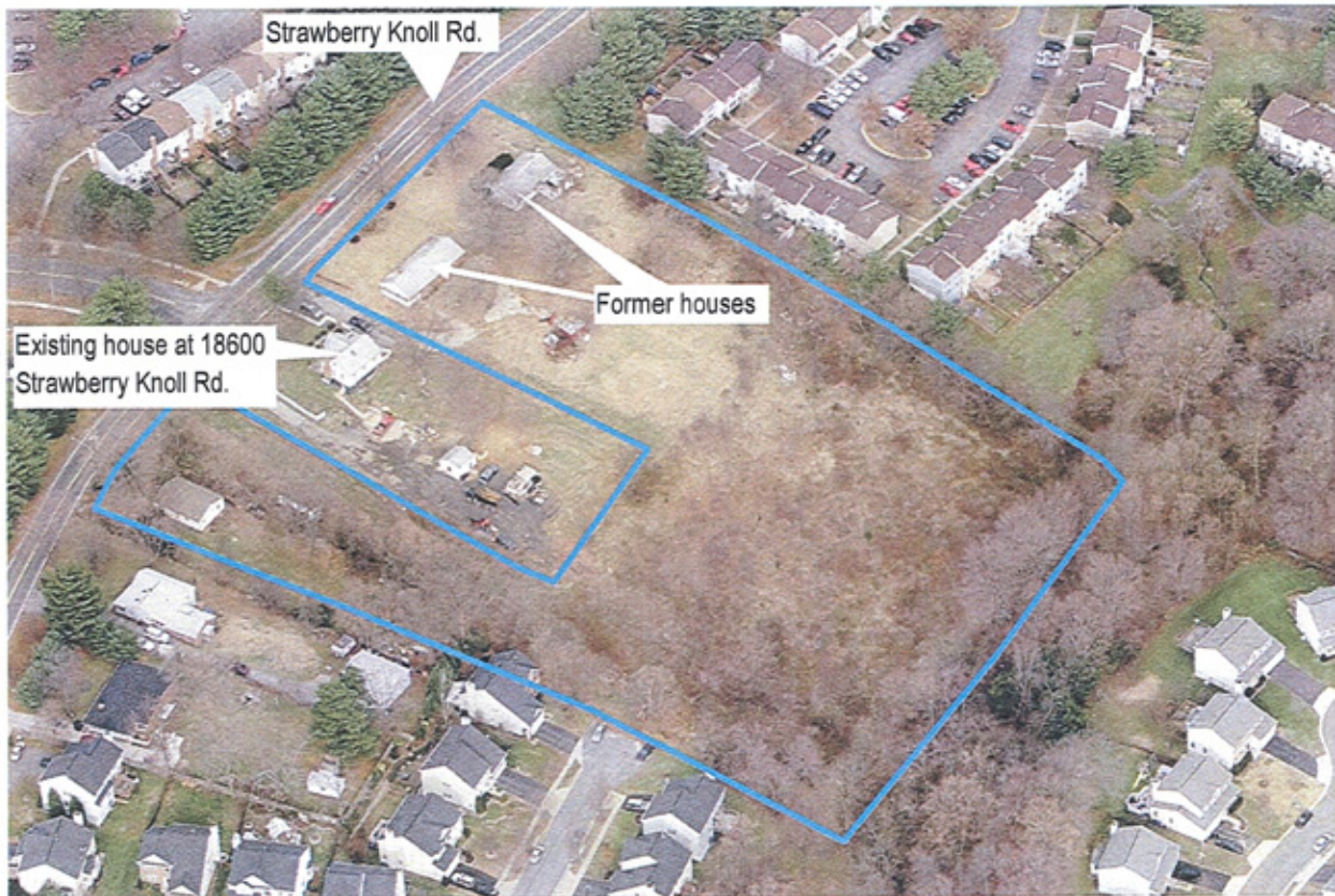
Aerial Photo with approximate site boundary outlined in blue
