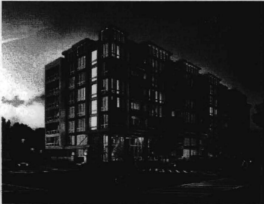
View of Southeast Corner of Building
