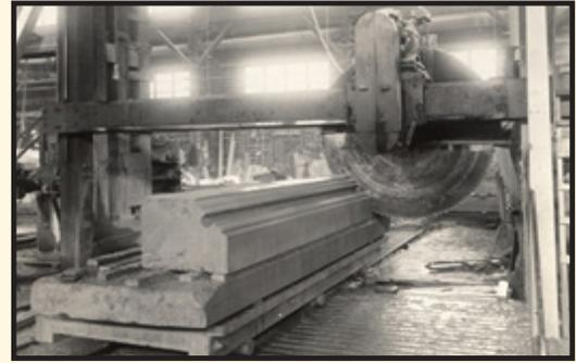
*Large stone-cutting machine at Fuller Plant*
