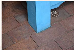
Hinge post set into masonry
