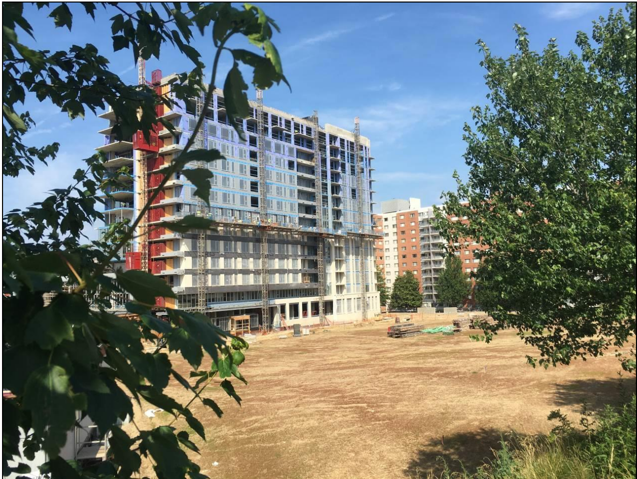
Figure 2 - Existing Site Conditions
