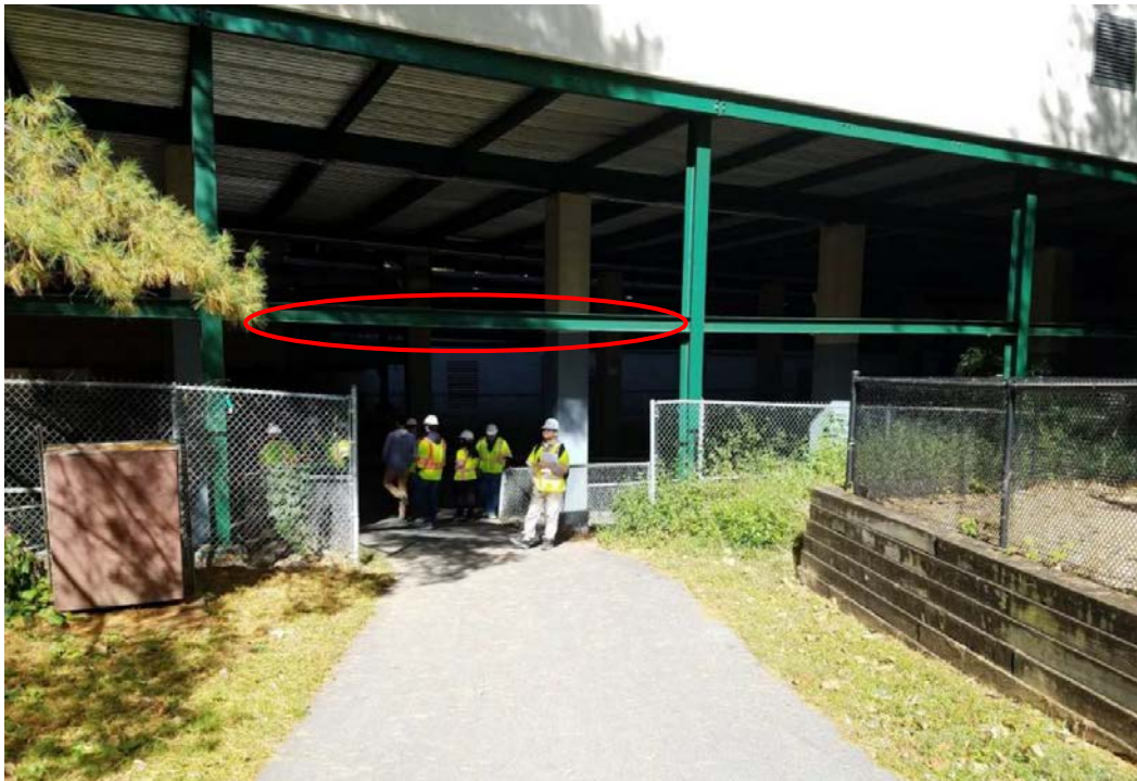
Horizontal beam supporting the Air Rights Building Parking Garage
