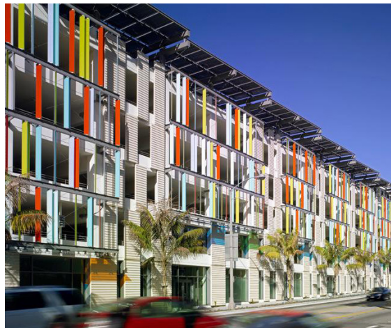
Parking garage with ground floor liner and a well composed architectural facade with shading and solar panels
