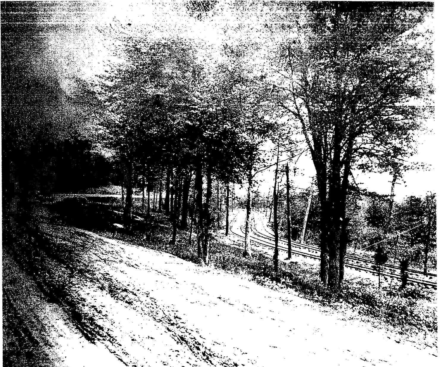
Figure 17. The Washington and Glen Echo Trolley tracks turn a curve just before the Sycamore Trestle and the Sycamore Stop. The old trolley right of way, and this curve in particular, are easily visible from MacArthur Boulevard driving inbound from the Clara Barton Parkway exit towards the Sycamore Store. Note that "Conduit Road" in the foreground is still a deeply tracked dirt road. Photo; courtesy of Montgomery County Historical Society.
